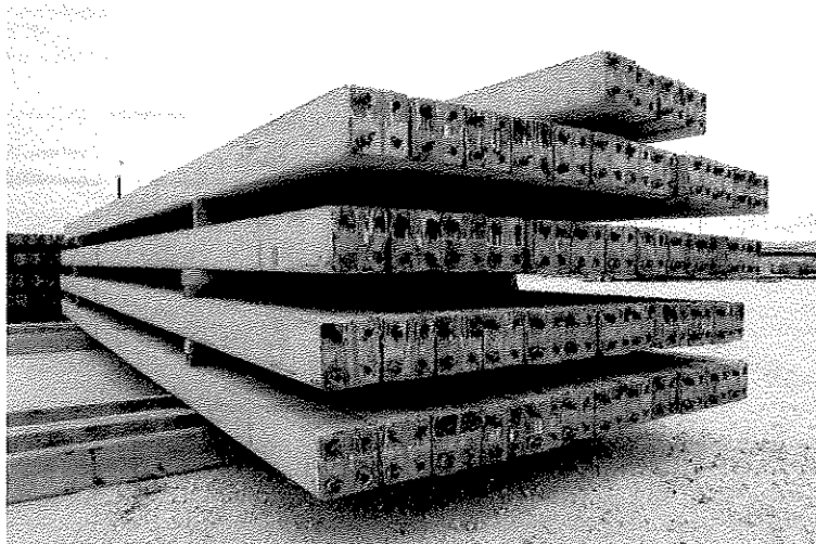
Stacked Piles to be Prepared for Driving
