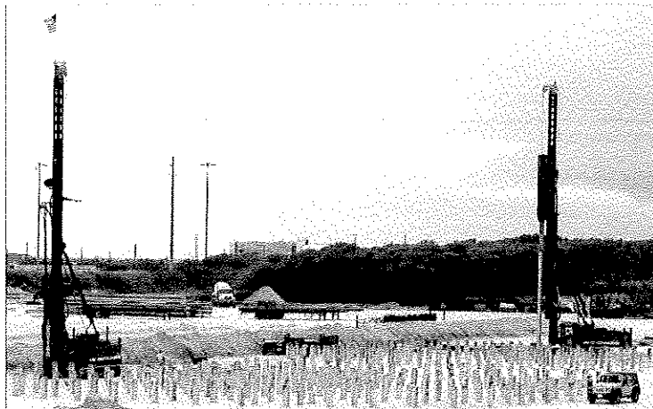
Driving Production Piles
