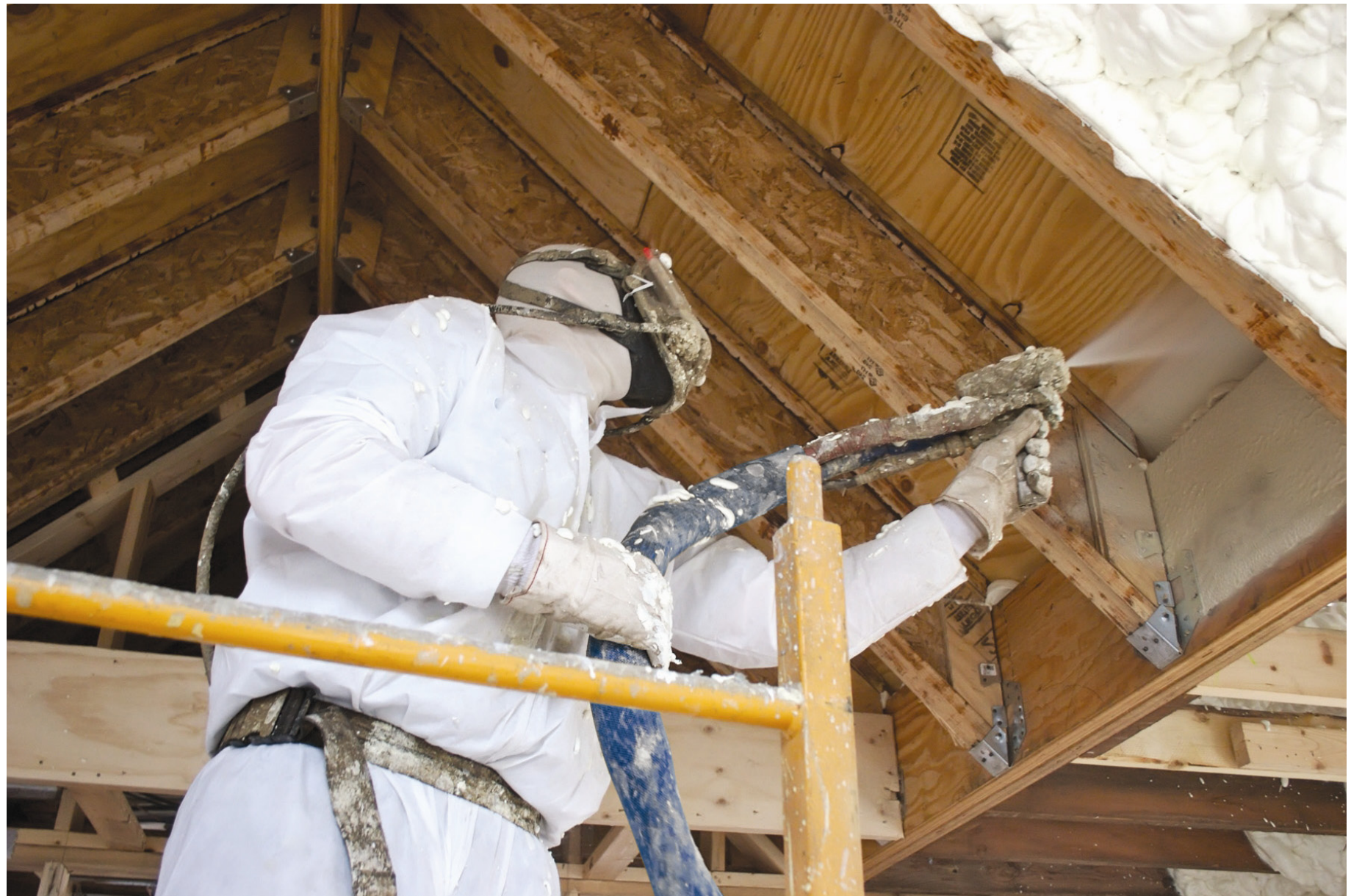
Application of SPF to the underside of sloped roof rafters.
