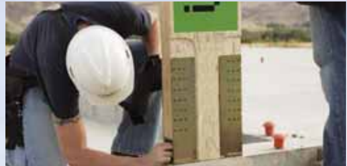
Shear Brace Portal Frame
