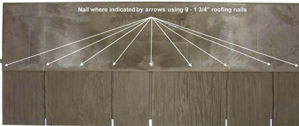
FIGURE 2—FASTENER LOCATIONS
