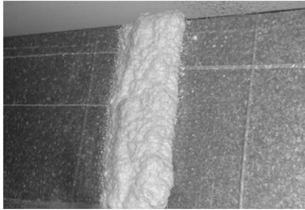
FIGURE 1—DUCT JOINT SEALING
